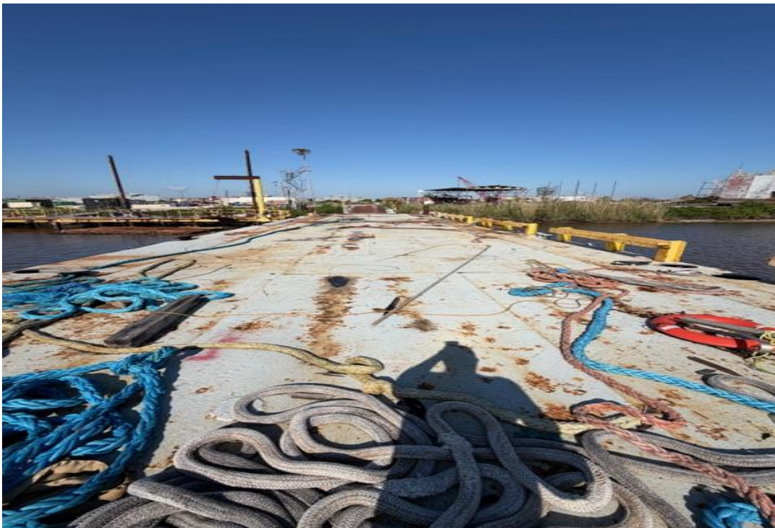
OVERALL VIEW OF DECK LOOKING AFT
