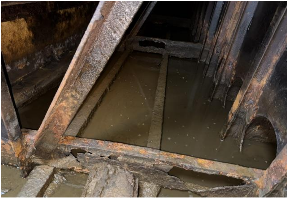
PORT NO. 2 CONTAINS HEAVY WASTAGE
